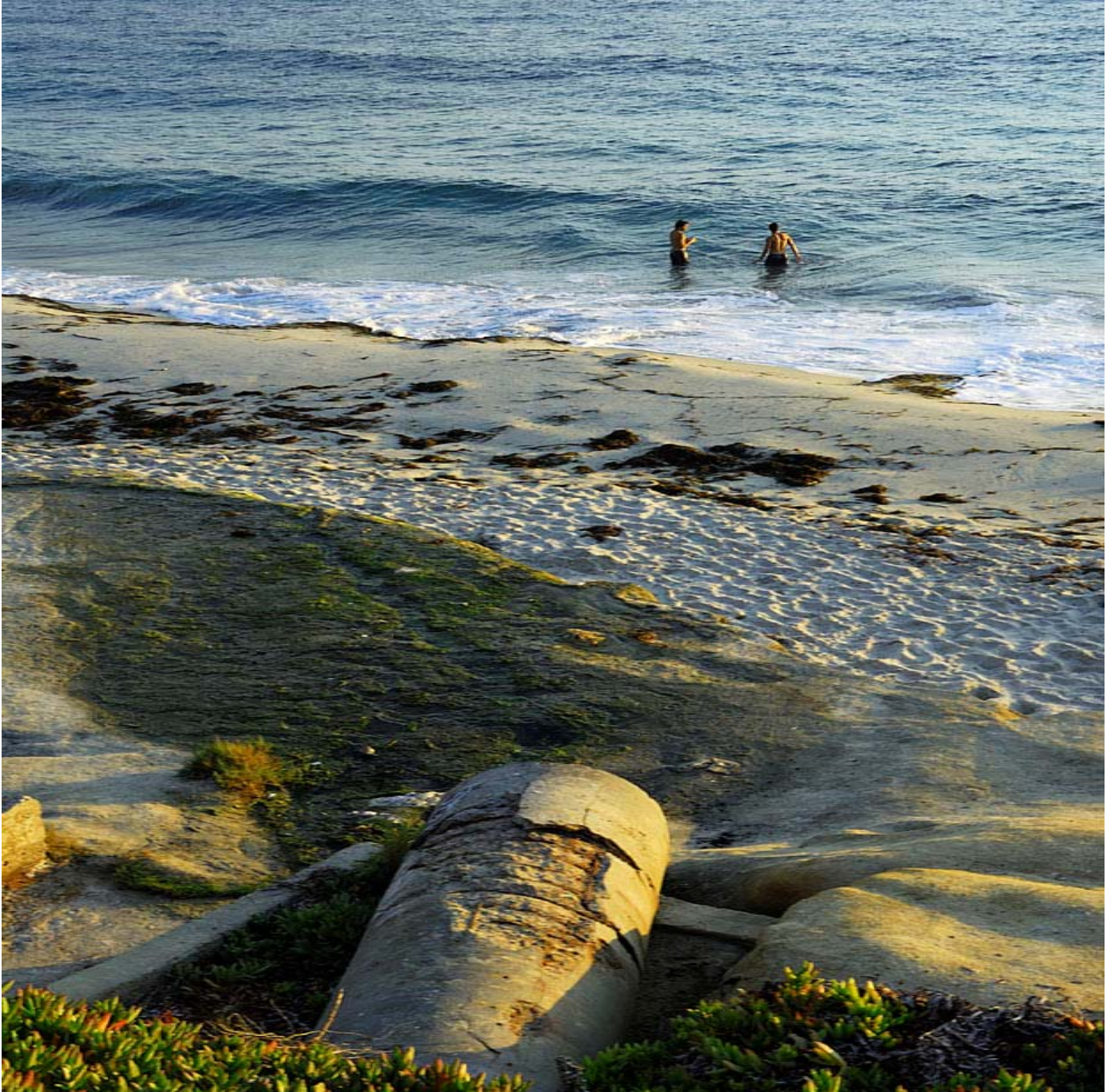
Figure A: Dry weather flow from a storm drain outlet at Windansea Beach in La Jolla. Photo: P. Neubauer
