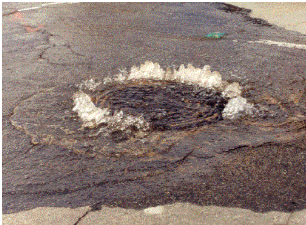
Figure 12: Sanitary sewer overflow (SSO)
